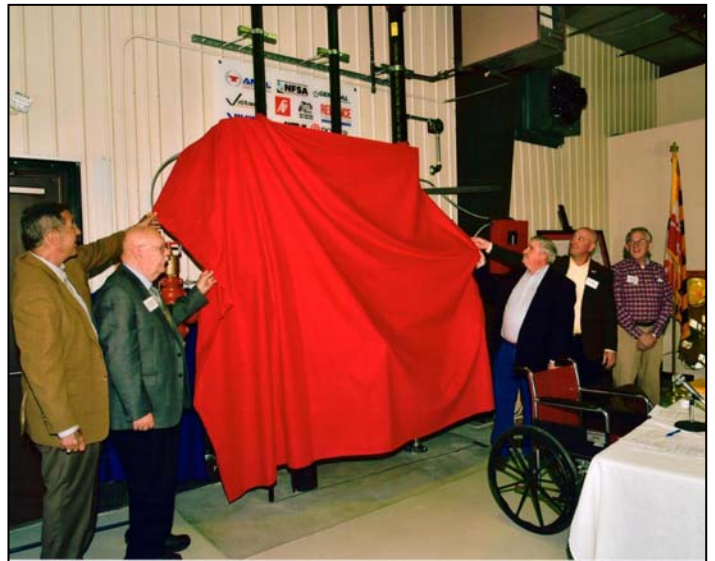
Unveiling the sprinkler system. (L-r) Jay Livingston, Ron Coleman, Terry Victor, Shane Ray, and Wayne Powell.
