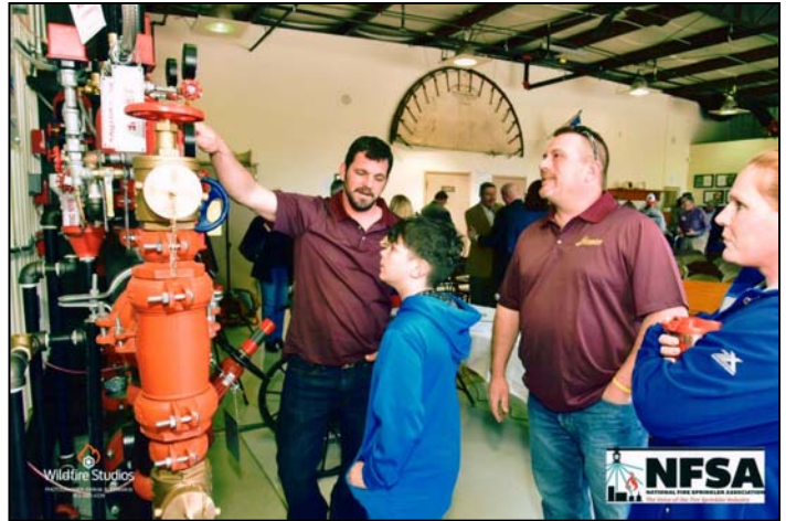
Learning about the sprinkler system - - - from some of the folks who installed it!
